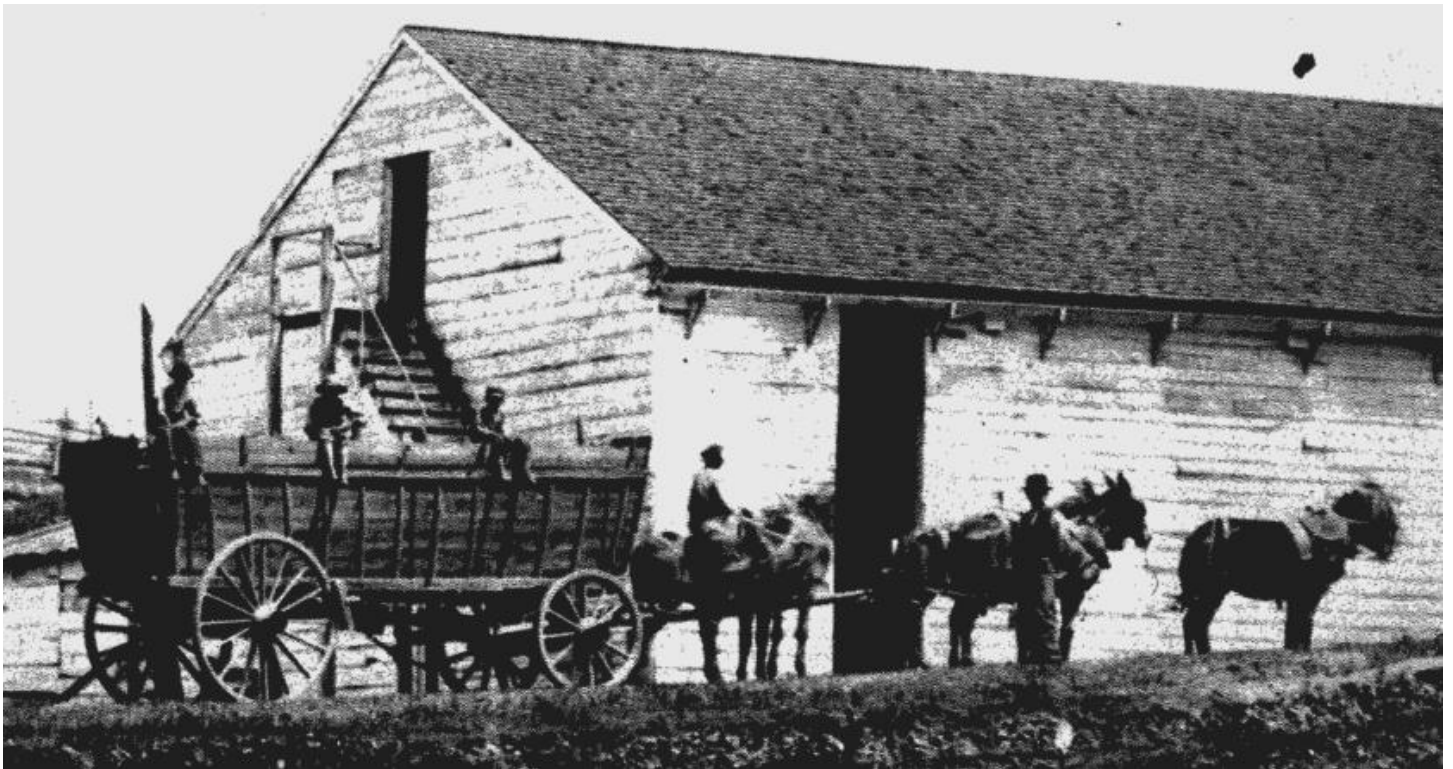
A typical wagon used to haul charcoal off the mountain, attached to a team of mules. Two adult teamsters are with the mules, and 3 boys can be seen sitting atop the wagon. The building is the Pine Grove Furnace “coal house” (it does not exist any longer). The top of the furnace stack is to the right of this view, probably taken around 1880.
