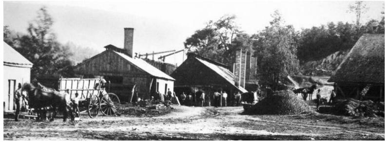
**Bottom: Laurel Forge dam after it failed in June 1889.** Horizontal logs in the “timber crib” are visible to left. The dam is missing in the middle. Note forge waterwheels.
